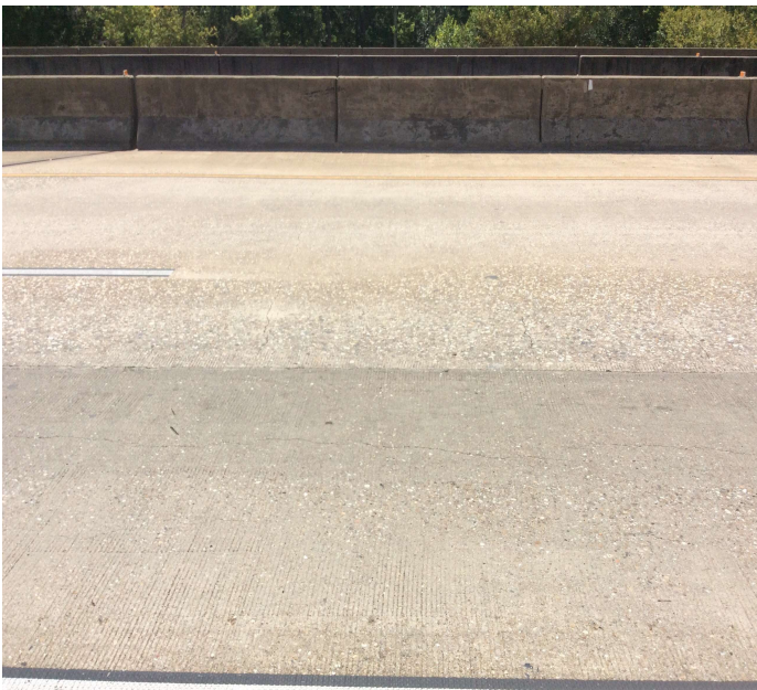
PHOTO 1 Description Span 8 deck has unsealed cracks.
