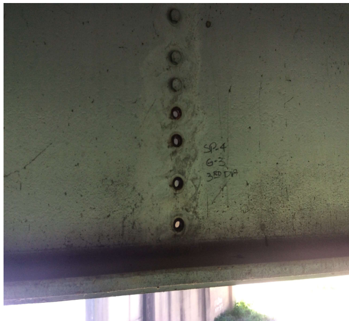
PHOTO 1 Description Span 4 beam 3 diaphragm 3 four missing bolts.
