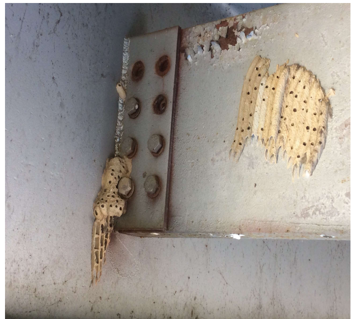
PHOTO 2 Description Span 5 beam 6 diaphragm 5 has missing and loose bolts.
