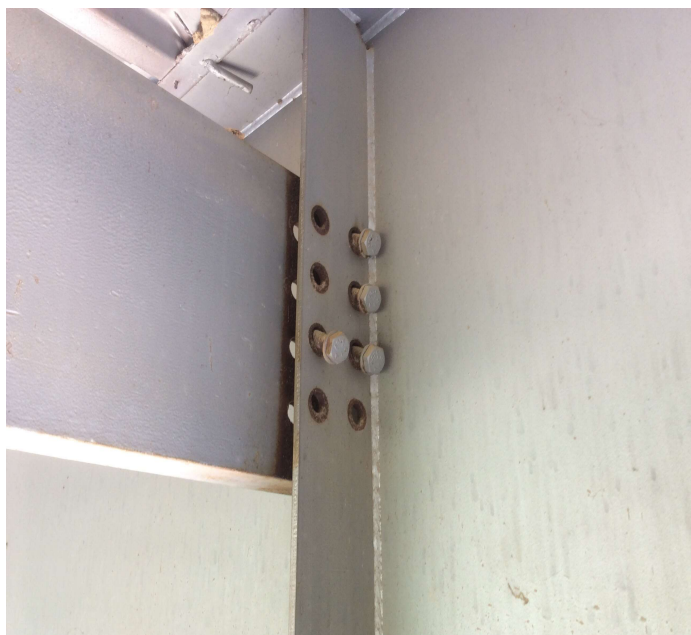
PHOTO 3 Description Span 10 beam 7 diaphragm 5 has missing and loose bolts.
