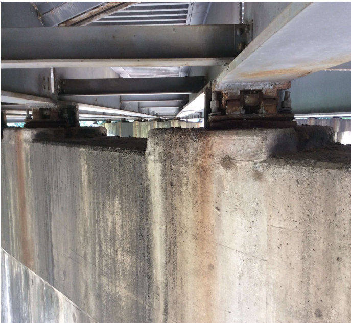
PHOTO 1 Description Bent 9 bearing have corrosion due to leaking joint seals. Common all bents.
